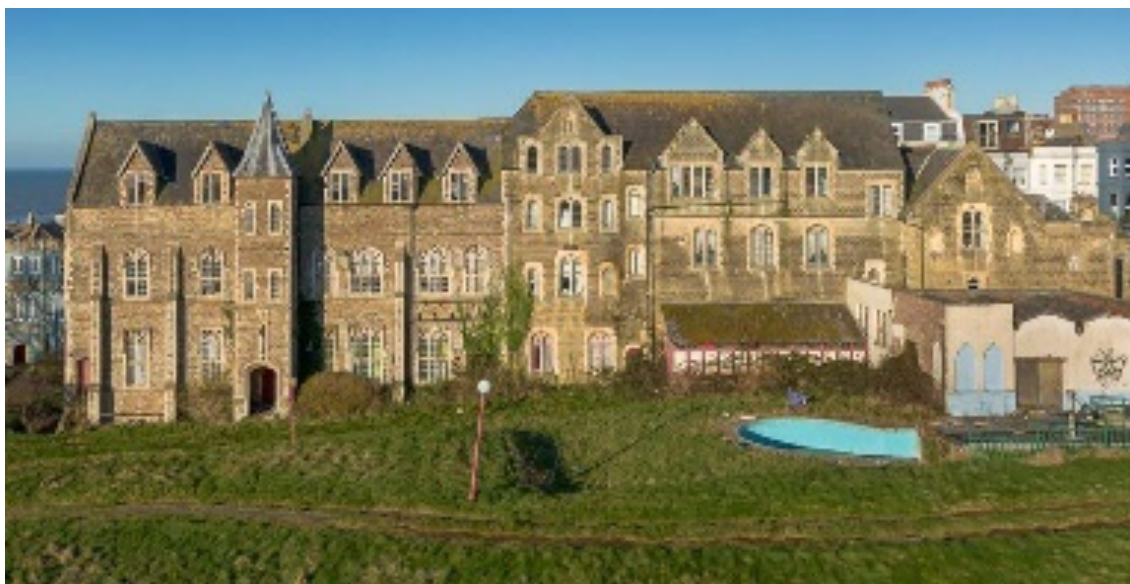
Site Photograph - East elevation of the Grade II listed Training College (Gothic Building) and Gate Lodge. Ref: Historic England, DP528338, 2025.
