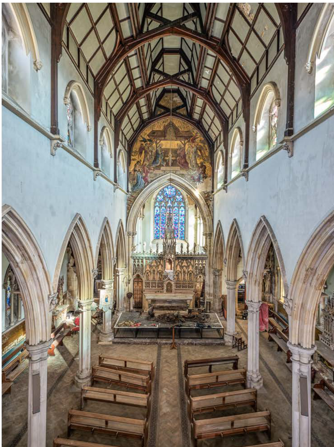
Site Photograph - De-consecrated former chapel, Grade II* listed.
