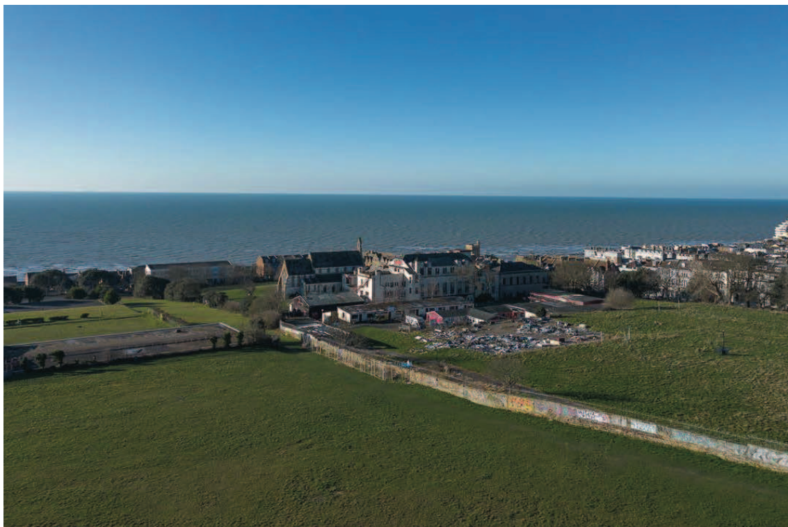
Site Photograph - North East - White Rock Gardens, parallel to Bohemia Road A21.
