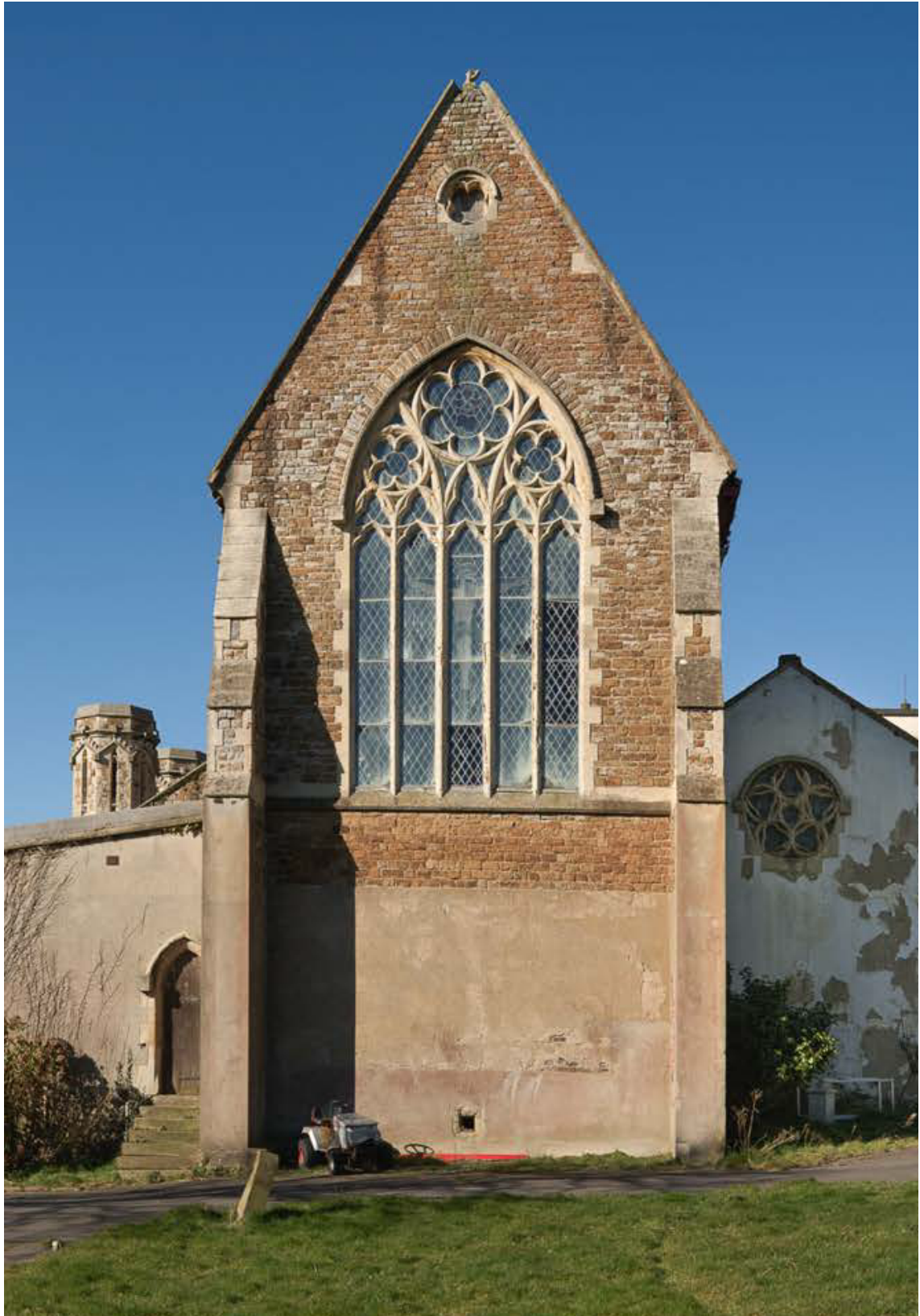
Site Photograph - Deconsecrated former chapel, Grade II* listed. Ref: Historic England, DP528359, 2025.
