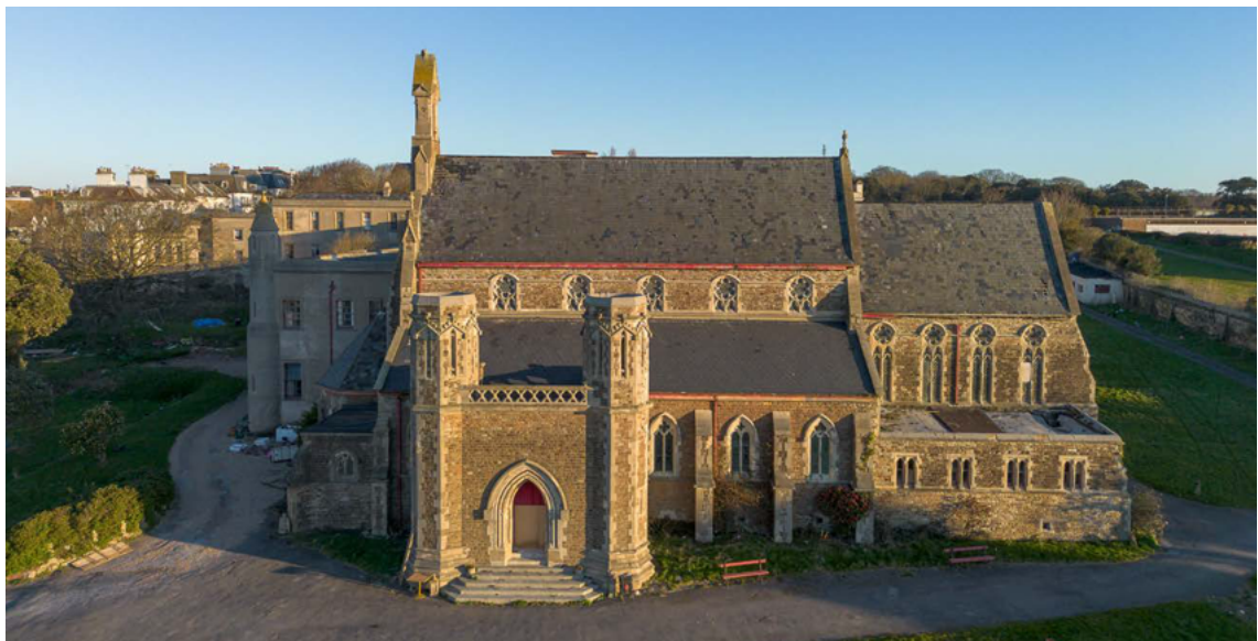
Site Photograph - Southern elevational view of the former chapel, with historic site photographs. Ref: Historic England, DP528364, 2025
