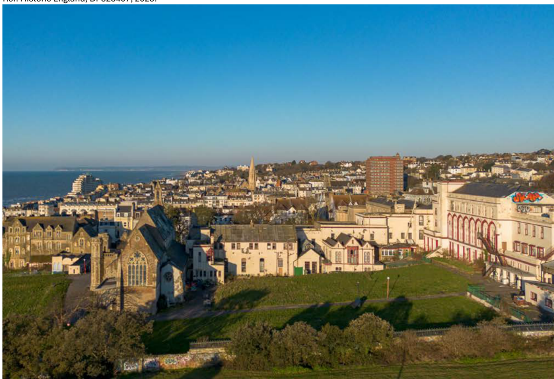
Site photograph - North East - White Rock Gardens, parallel to Hastings Skate Park.
