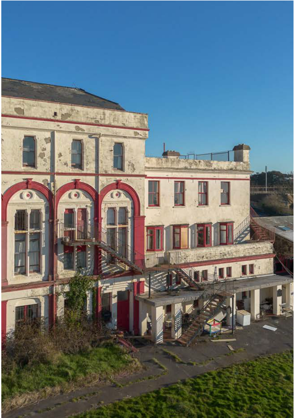
Site Photograph - 'New Building' a Pre-1948 curtilage listed building prior to the fire in July 2026.
